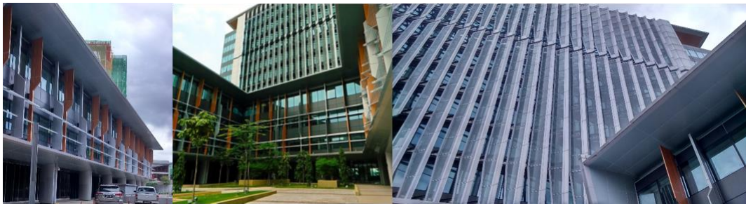
Fig. 4: Aluminium spandrel panels with horizontal aluminium louvers on N-S facades of low-rise (left), aluminium spandrel panels on E-W facades of low-rise (middle) and aluminium framed fritted glass fins on E-W facades of tower block (right) Source: Author
