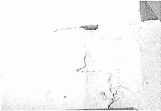
Figure 12 : Chipping of defective plaster on wall
