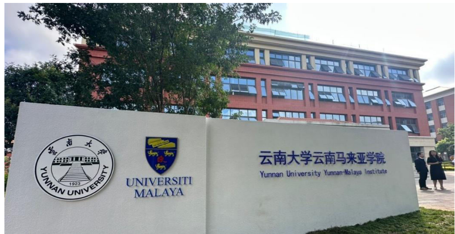
One of three newly-constructed buildings that make up the Yunnan-Malaya Institute.
